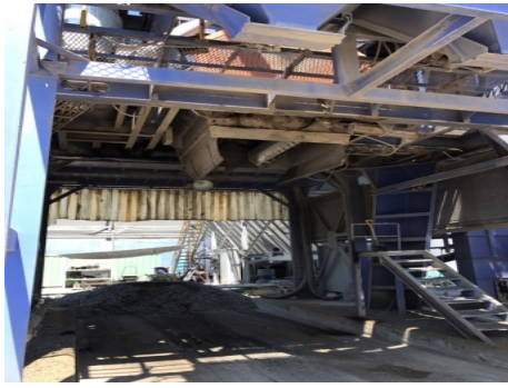
<Ascon mixing machine>
